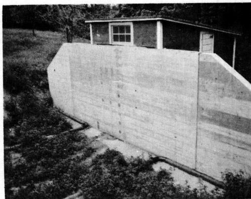
Figure 14. Rehabilitated retaining wall with pressure cells installed - 1952.
