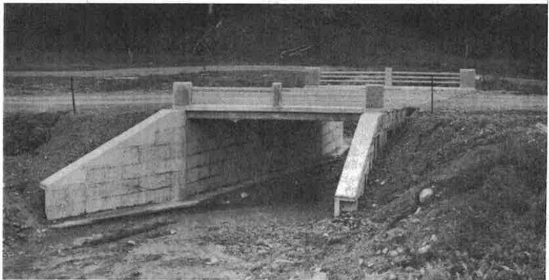
Figure 4. Bridge No. 14, Perry, Wyoming County, New York.
