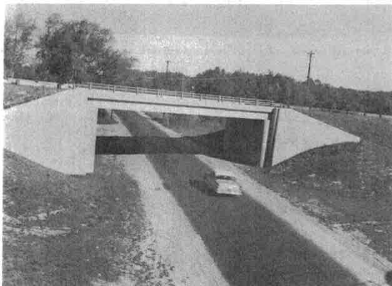
Figure 10. Single-span prestressed bridge over Route 559, Garden State Parkway bridges, Section II.
