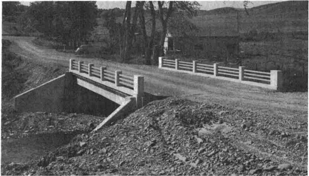
Figure 3. Bridge, No. 7, Pike, Wyoming County, New York.
