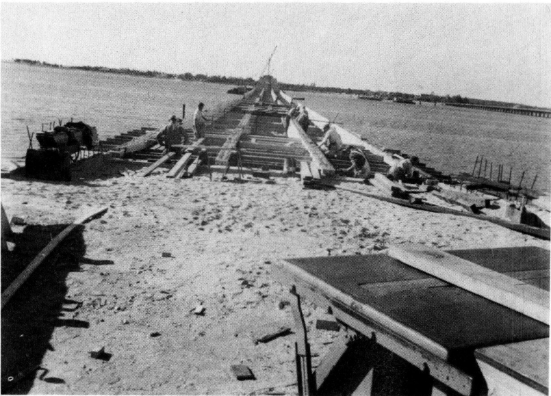
Figure 15. Great Egg Harbor Bay Bridge (looking south). Deck slab forms being erected, Garden State Parkway, N.J.
