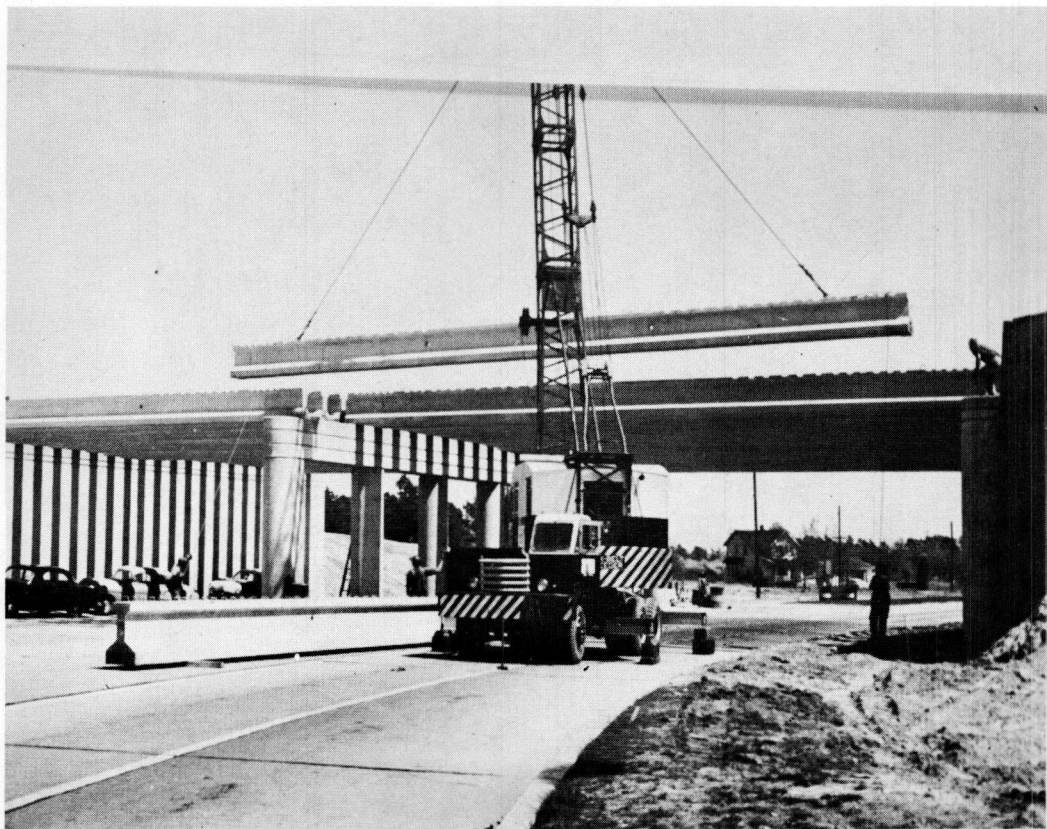
Figure 8. Prestressed beams erected at site over US 322, Garden State Parkway bridges, Section II.
