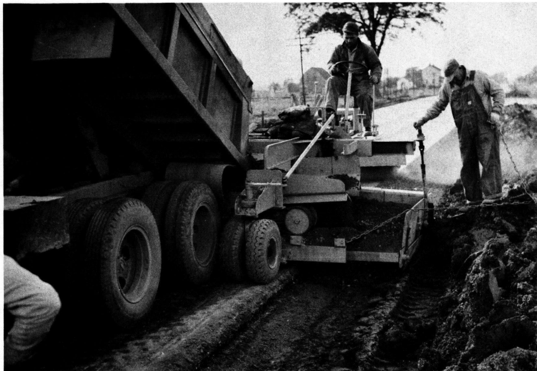
Figure 6. Stabilized crushed aggregate shoulder material being placed with mechanical spreader.
