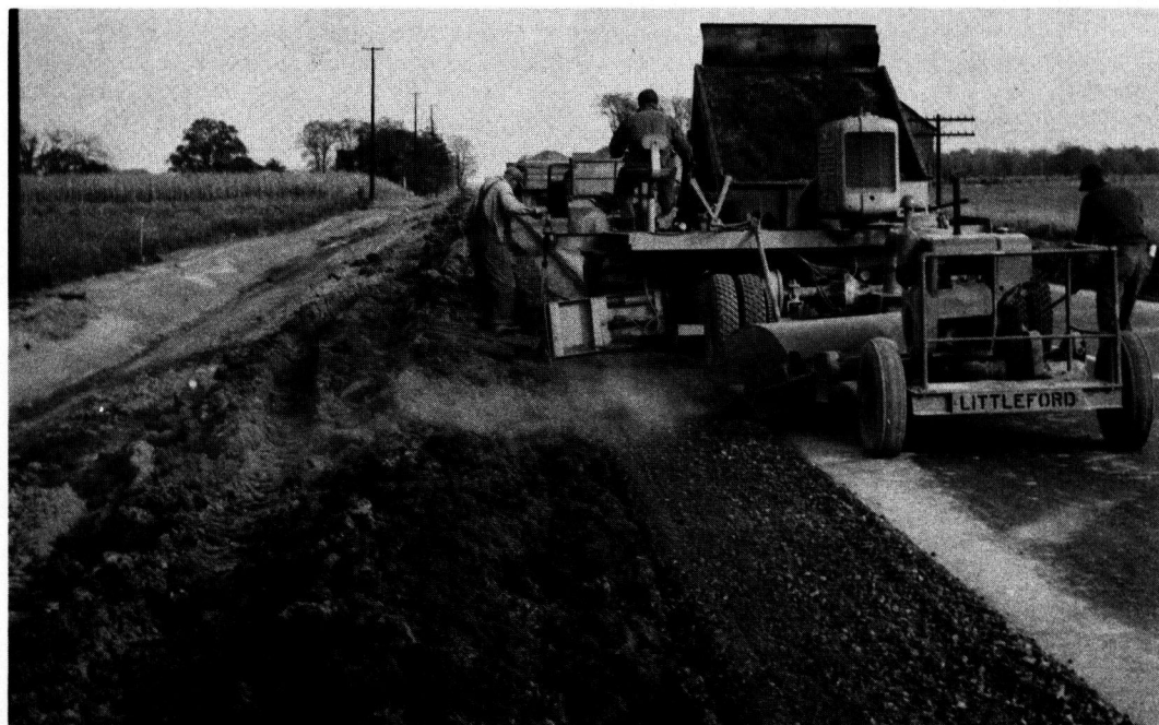
Figure 7. Rear view of spreading operation, showing towed power broom being used to keep pavement clean and free from loose aggregate.
