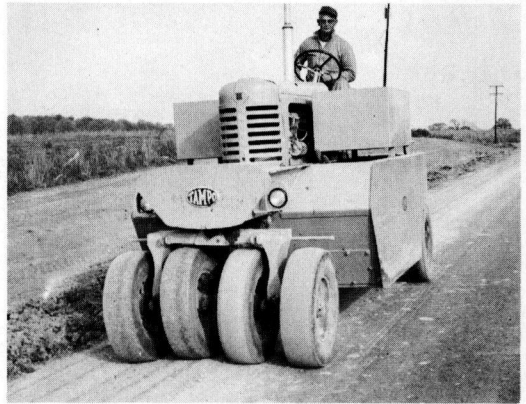
Figure 8. Pneumatic tired roller being used to compact stabilized crushed aggregate shoulder.
