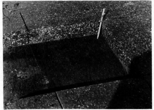
Figure 5. Outer block removed from pavement.
