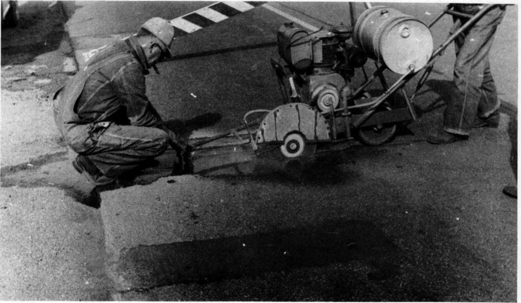
Figure 3. Sawing specimens from the highway.
