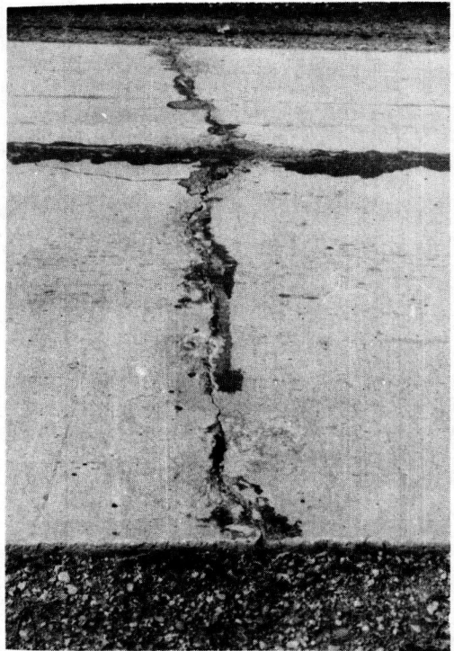
Figure 9. Typical of the cracks occurring in the plain concrete sections (Designs 5, 6, 10 and 10-Tar Paper) and which shows a normal amount of concrete disintegration associated with most cracks in these sections. Faulting is also characteristic of most of these cracks.
