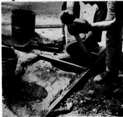
FIGURE 15. ADDING GROUTING MIXTURE.
