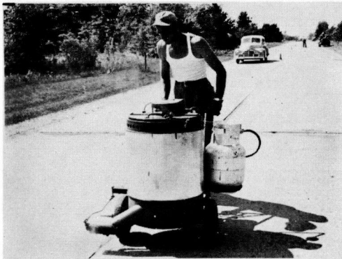
FIGURE 2. SEALING LONGITUDINAL JOINT WITH MECHANICAL POURPOT.
