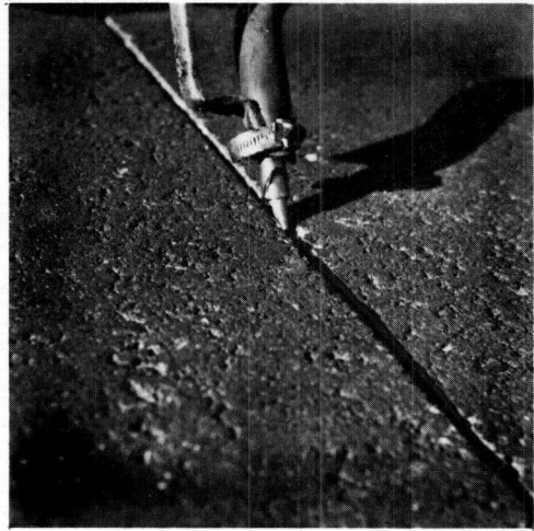
Figure 12. Cold-applied materials were placed under pressure.
