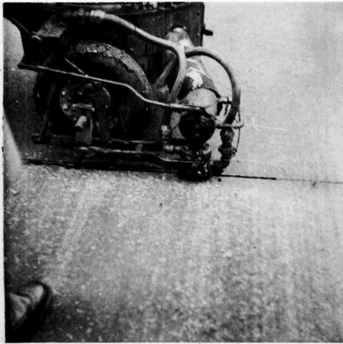
Figure 11. Hot-poured materials were applied with double boiler applicator.
