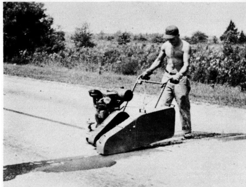
FIGURE 3. CONTRACTOR'S JOINT - CLEANING MACHINE IN OPERATION.
