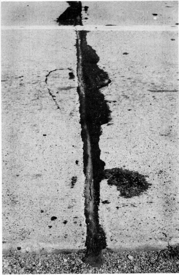
FIGURE 24. TYPICAL OF SURFACE CRACKING AND WRINKLING OF BRAND C AT 3 YEARS. SEAL STILL INTACT.
