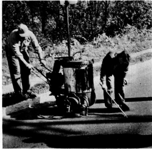
Figure 3. Sealing a crack with a hot-poured material.
