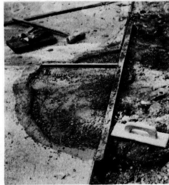
FIGURE 16. READY FOR FINISH COAT.
