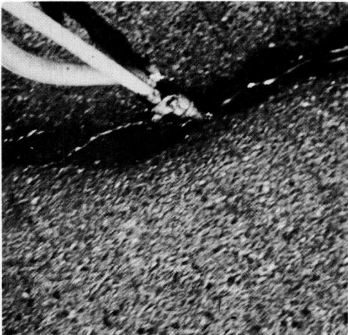
Figure 20. Experimental sealing machine. Sealing nozzle in operation.
