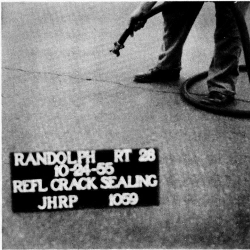
Figure 2. Air blowing a crack before sealing.
