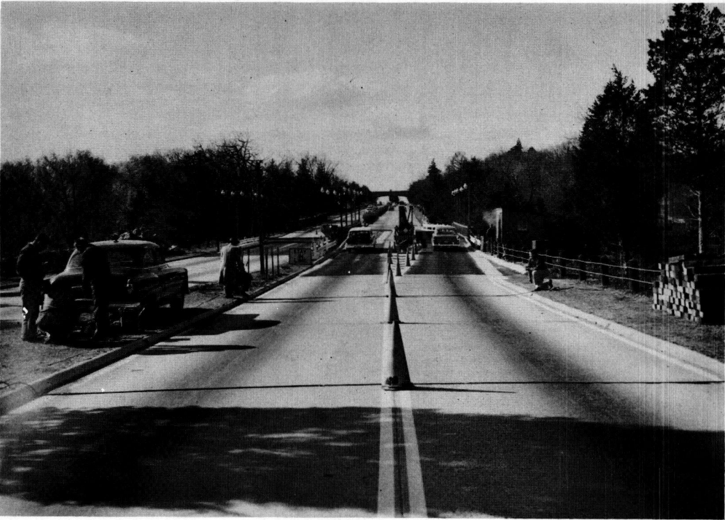
Figure 1. Temporary bridge site (as seen by westbound traffic).
