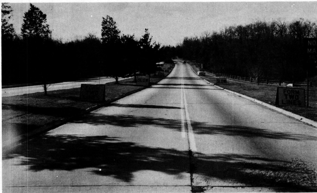
Figure 3. Signing program - approaching temporary bridge.
