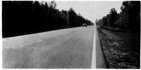
Figure 3. Study location No. 1—(a) Normal, with centerline only; (b) Continuous stripe 18 in. from edge of pavement.
