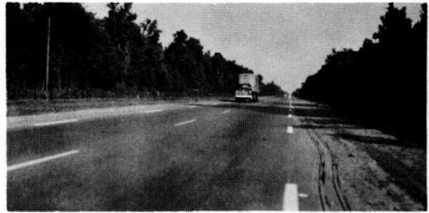
Figure 4. Study location No. 2—(a) Normal, with centerline only; (b) 10 ft stripe 12 in. from edge of pavement.
