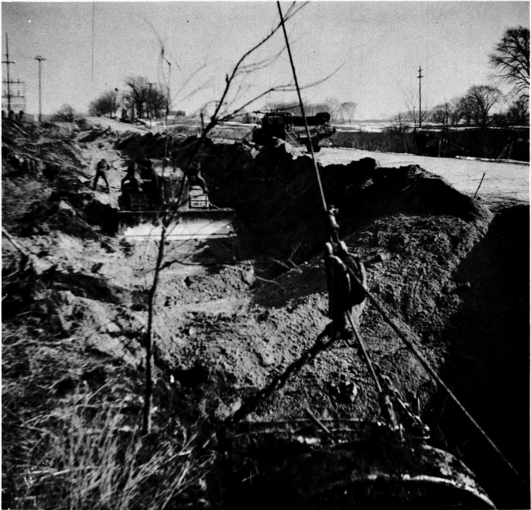
Figure 2. Typical muck excavation and backfill with selected material.
