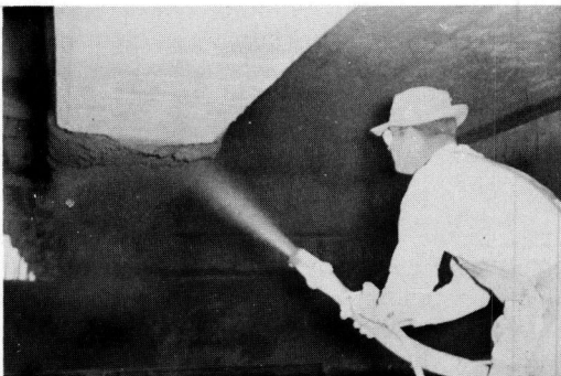
Figure 15. Nozzlemán "shooting" beam requiring repair through part of its length.
