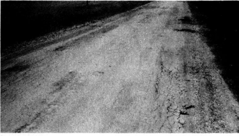
Figure 1. Typical surface condition prior to stabilization.
