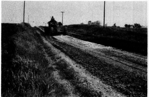
Figure 6. Mixing base materials and sodium chloride.
