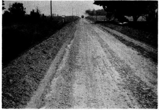
Figure 4. Existing base material windrowed to sides.
