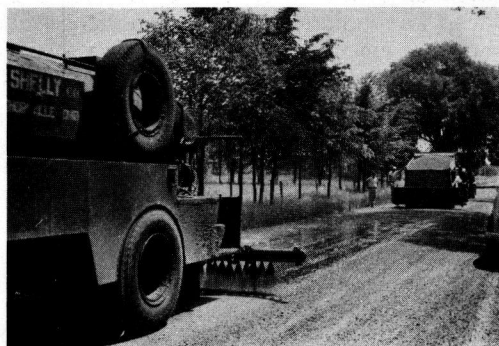
Figure 11. Applying bituminous prime and cover chips.
