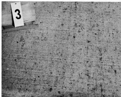
Figure 4. Passing lane of a concrete pavement constructed in 1951 with relatively little accumulation of oil droppings.
