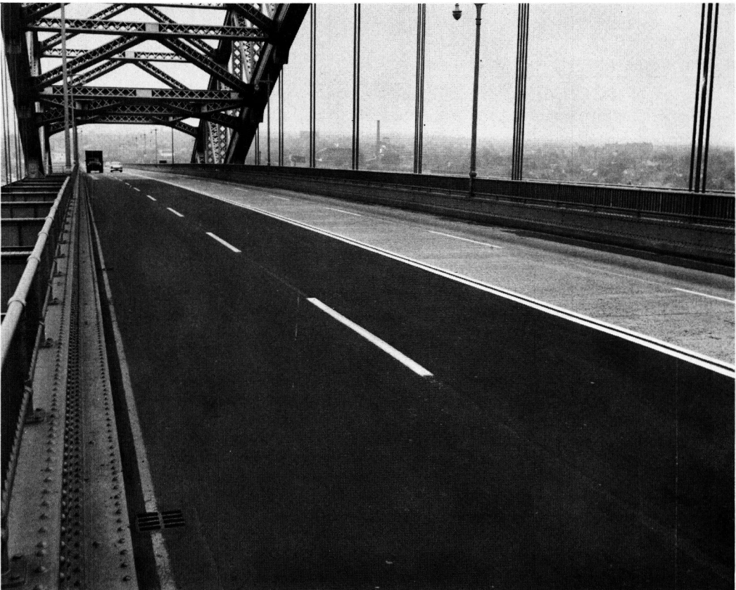
Figure 3. Bayonne Bridge, test section of silica sand asphalt after 10 months of service 7,000 cars per day.
