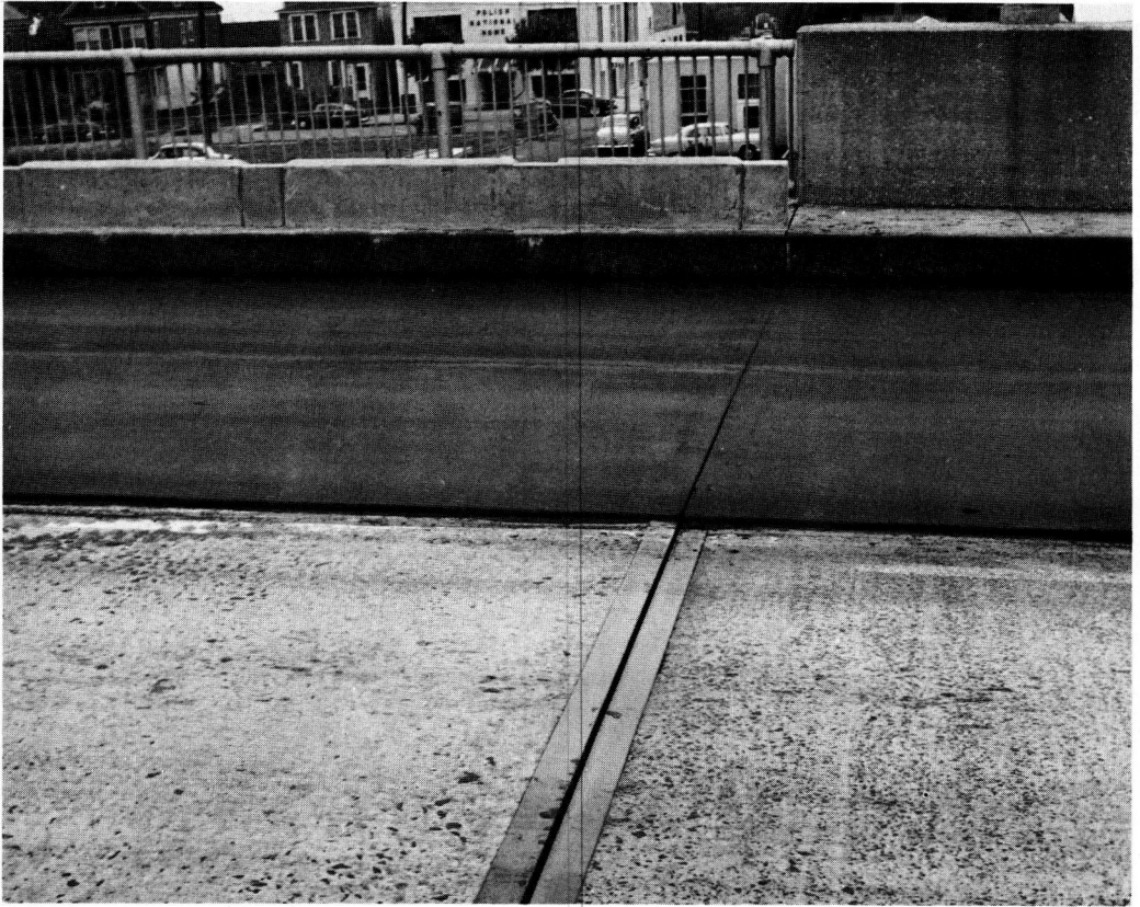
Figure 8. Goethals Bridge, 1/2 in. silica sand asphalt resurfacing at abutment joint.
