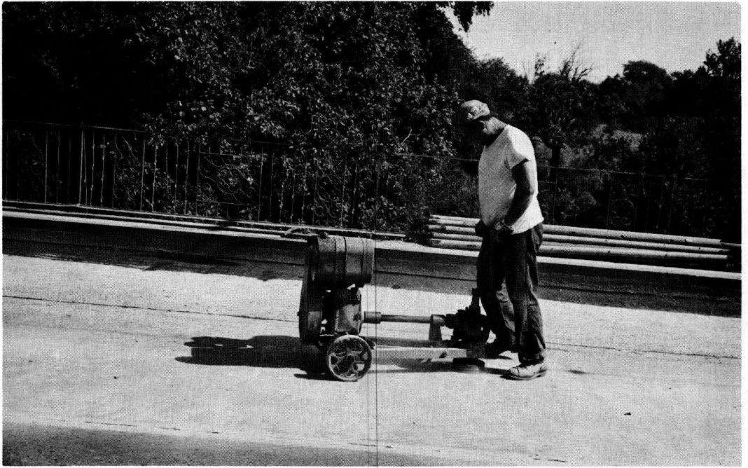
Figure 1. Removal of heavy tar and grease spots.
