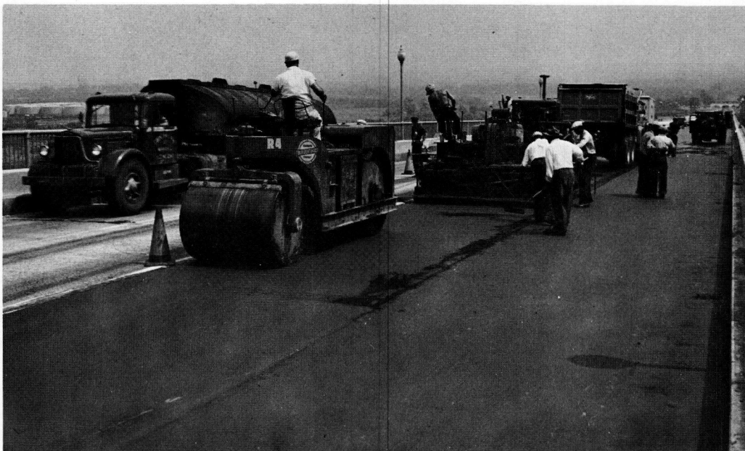
Figure 6. Goethals Bridge, laying silica sand asphalt \frac{1}{2} in. thick using standard asphalt equipment.
