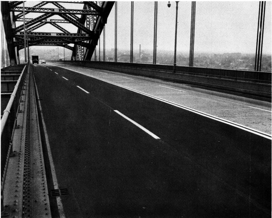
Figure 3. Bayonne Bridge, test section of silica sand asphalt after 10 months of service 7,000 cars per day.
