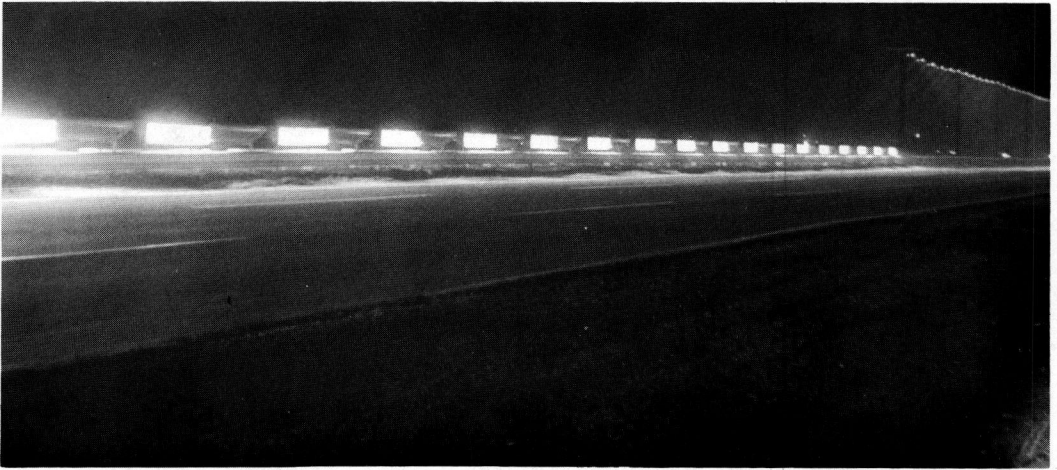
Figure 10. Low mounted fluorescents installed on the New Jersey Turnpike. These are 8 ft, 200 w. lamps, 18 ft on centers, mounted just above the guardrails. The reflectors direct the light below the horizontal. Louvres are used to reduce the component toward oncoming traffic.
