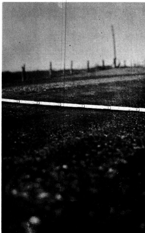
Figure 6. Quicklime, Section II, distortion in outer wheel track.
