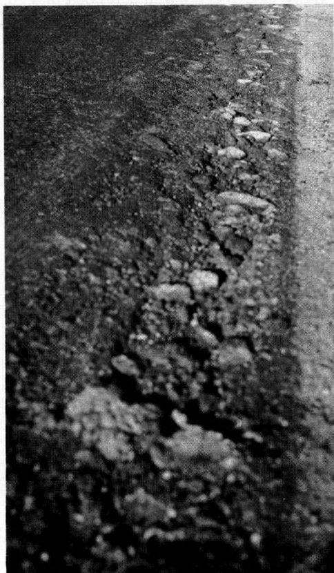
Figure 8. Waste lime, Section II, edge distress.
