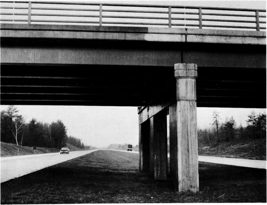
Figure 11. Close-up of pier facing and fascia (November 28, 1957).
