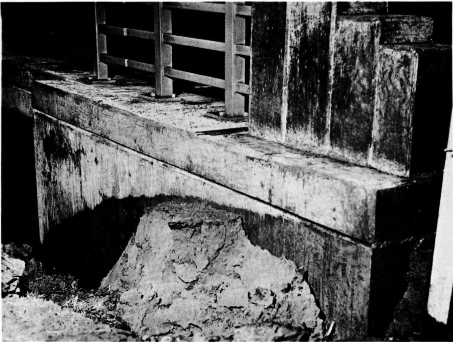
Figure 12. Carborundum rubbed pylon exhibits very little benefit from treatment.
