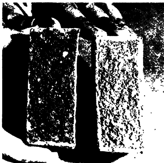
Figure 1. Depth of penetration of silicone in mortar block on right and concrete block on left.
