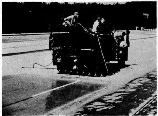
Figure 7. Equipment for spraying silicone solution on traveled way.
