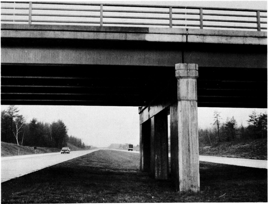
Figure 11. Close-up of pier facing and fascia (November 28, 1957).
