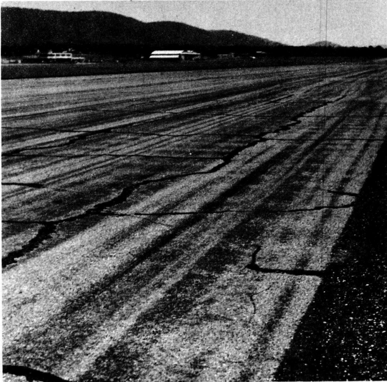
Figure 1. Typical cracking pattern.
