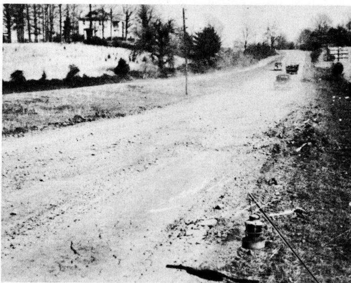
Figure 6. Failure of A Primary Highway (Surface Treated Water-Bound Macadam) - Rt. 29, Culpeper County - This portion of the road is located in Triassic "Red Bed" soil area. Approximately 60 percent of the primary roads in this soil area were rated as poor at the time of the spring break-up.
