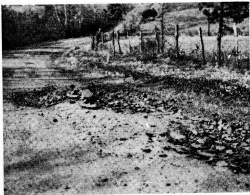
Figure 12. Distress of a Surface Treated Mechanically Stabilized Base Secondary Road - Rt. 609, Culpeper County.
