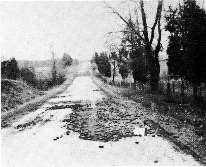
Figure 9. Alligator Cracking and Disintegration of Surface Treated Selected Soil Base Road in High-Quartz Granitoid Soil Area - Rt. 3, Orange County. Because of their high silt content these soils are subject to frost action.
