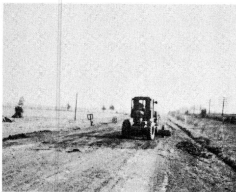
Figure 6. Failure of A Primary Highway (Surface Treated Water-Bound Macadam) - Rt. 29, Culpeper County - This portion of the road is located in Triassic "Red Bed" soil area. Approximately 60 percent of the primary roads in this soil area were rated as poor at the time of the spring break-up.
