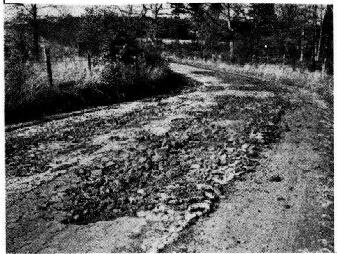
Figure 11. Excellent Performance of a Surface Treated Macadam Base Secondary Road, Rt. 627, Orange County.
