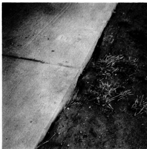
Blowing along edge--at joint and near mid-slab.
