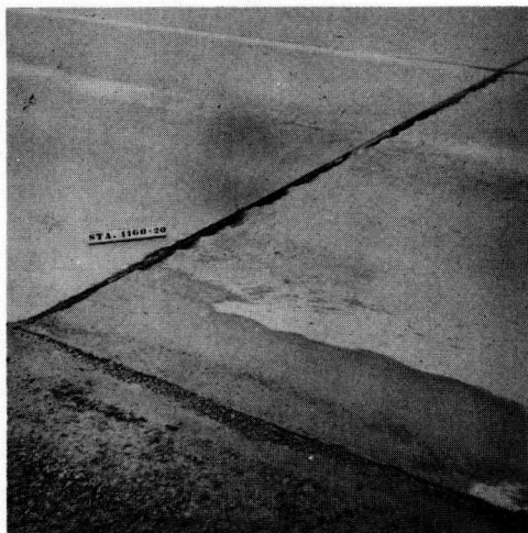
Examples of pumping at joint and edge.
