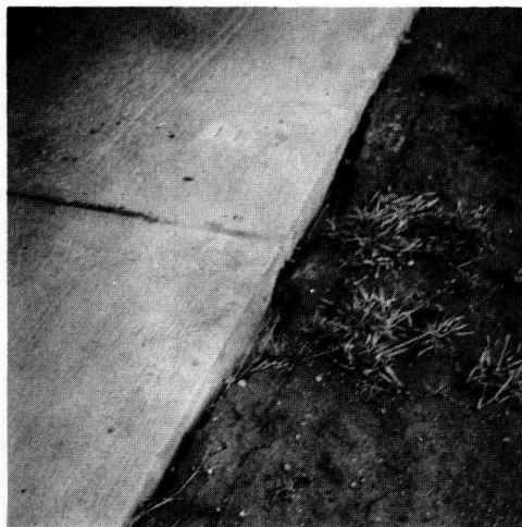
Blowing along edge--at joint and near mid-slab.
