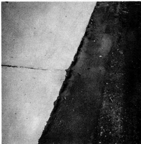
Examples of pumping at joint and edge.
