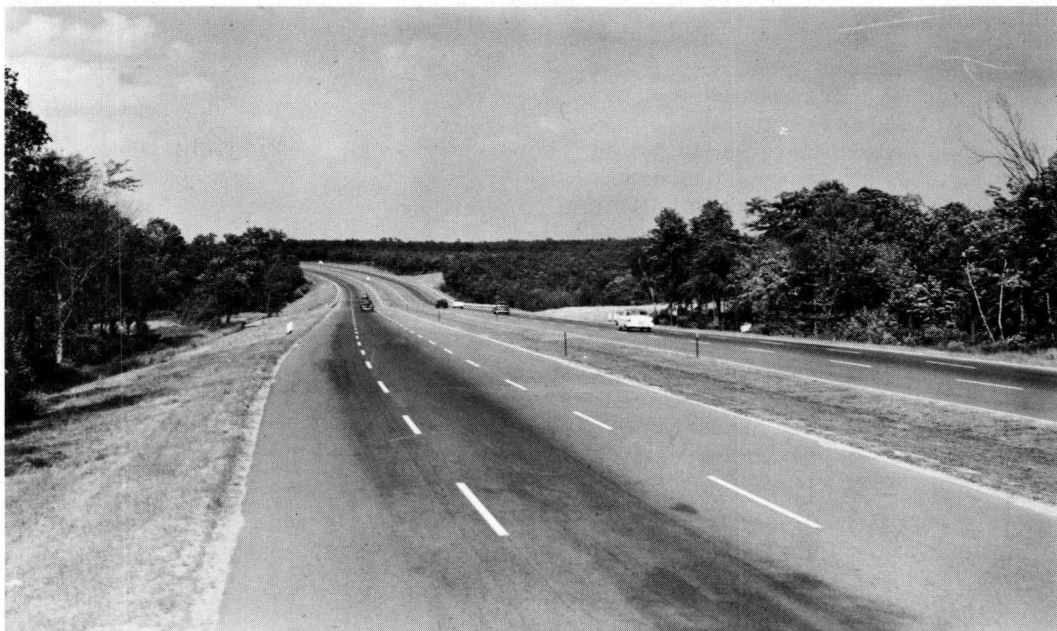
Figure 3. Fall River Expressway between Taunton and Fall River, Massachusetts—Right-of-way costs will be reduced by advance acquisition of land.
