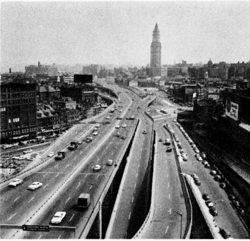
Figure 1. John R. Fitzgerald Expressway, Boston, Massachusetts—Many aspects of expressway law were involved in connection with this modern expressway running through the center of the city.
