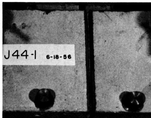
Figure 6. Cohesion failure of polysulfide rubber.
