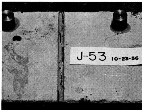
Figure 7. Failure of modified epoxy sealer in both adhesion and cohesion.
