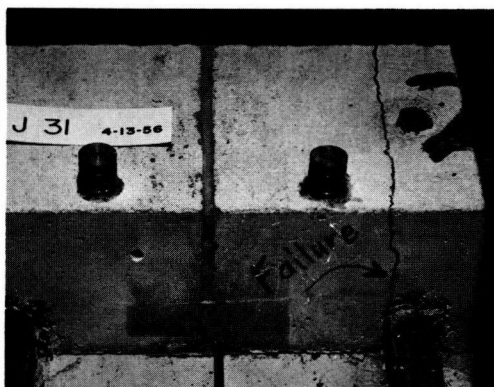
Figure 8. Failure of concrete resulting from high tensile bond strength and high tensile modulus of urethane sealer.
