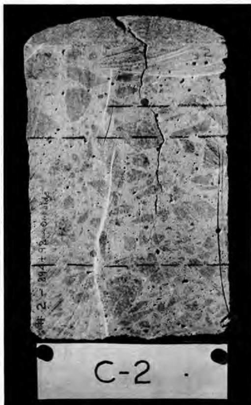
Figure 12. Core at crack in 10-in. section, Sta. 894+92.
