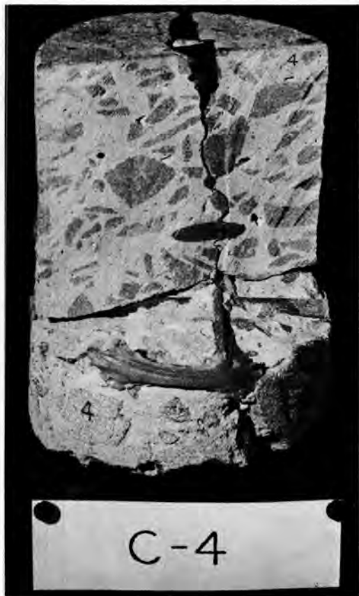
Figure 18. Core at crack near construction joint, 8-in. section.
