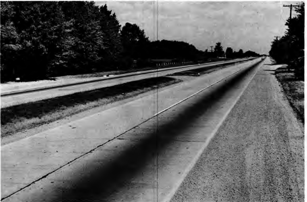
Figure 2. Eight-inch section looking north.
