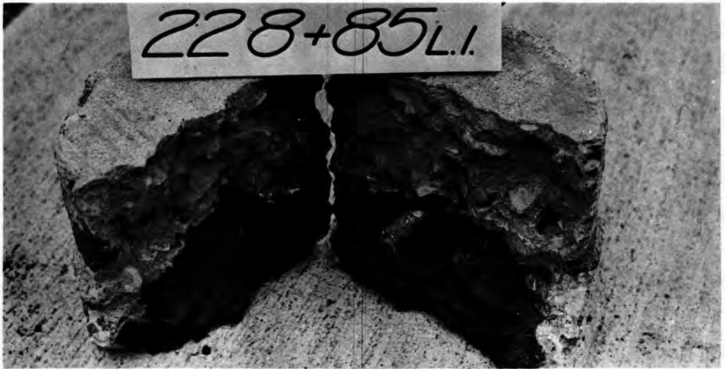
Figure 12. Separate halves of core at station 228+85.
