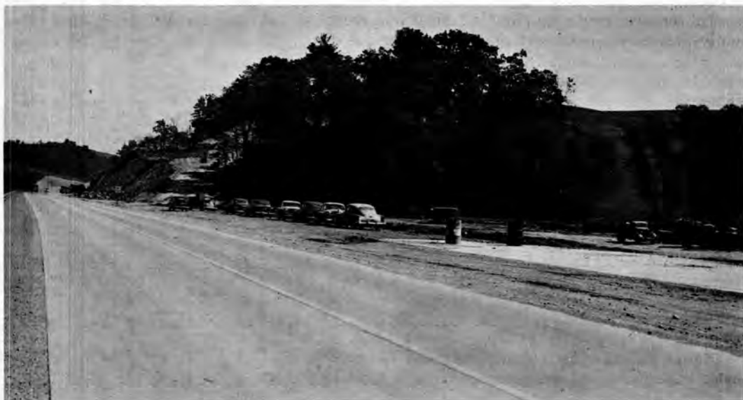
Figure 2. Slide area near Station 246, eastbound lanes.
