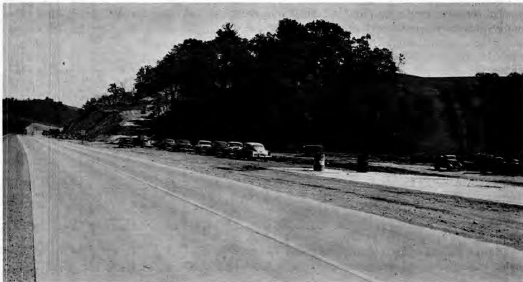
Figure 2. Slide area near Station 246, eastbound lanes.
