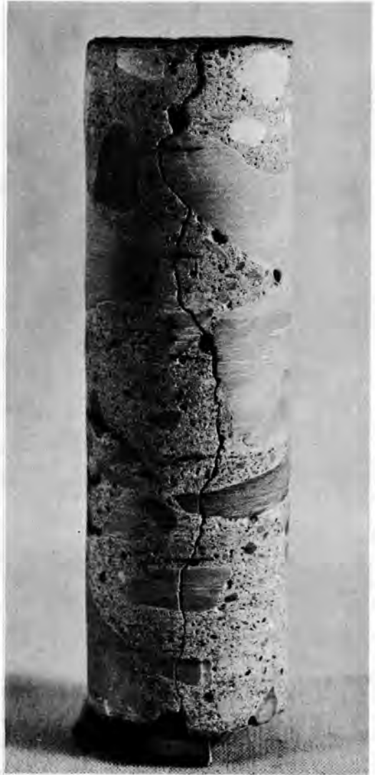
Figure 7. Core through representative transverse crack in 7-in. pavement with 0.3 percent steel.
