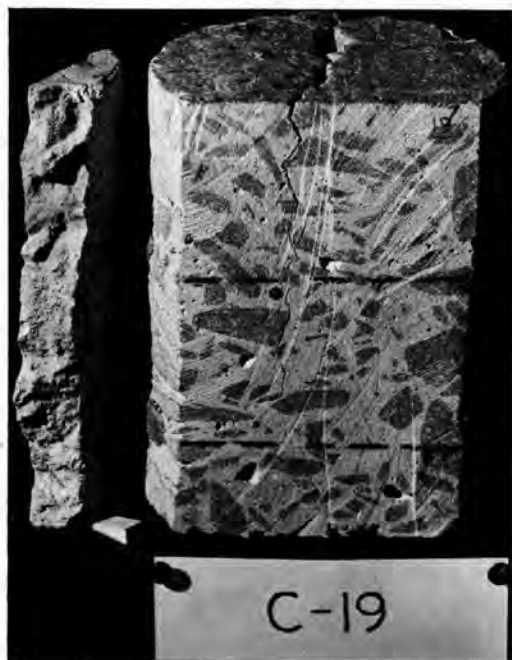
Figure 17. Core at crack in 8-in. section, Sta. 823+08.
