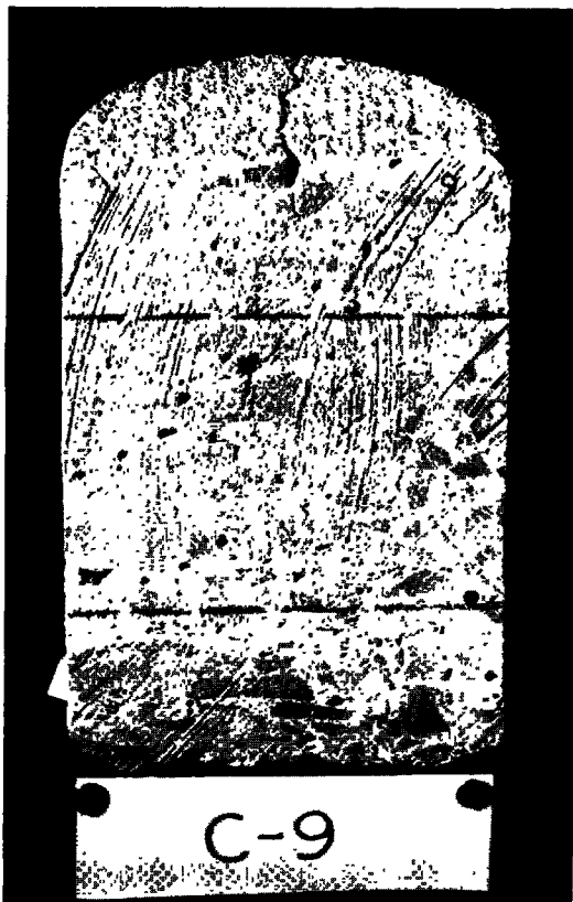
Figure 14. Core at crack in 10-in. section, Sta. 894+88.
