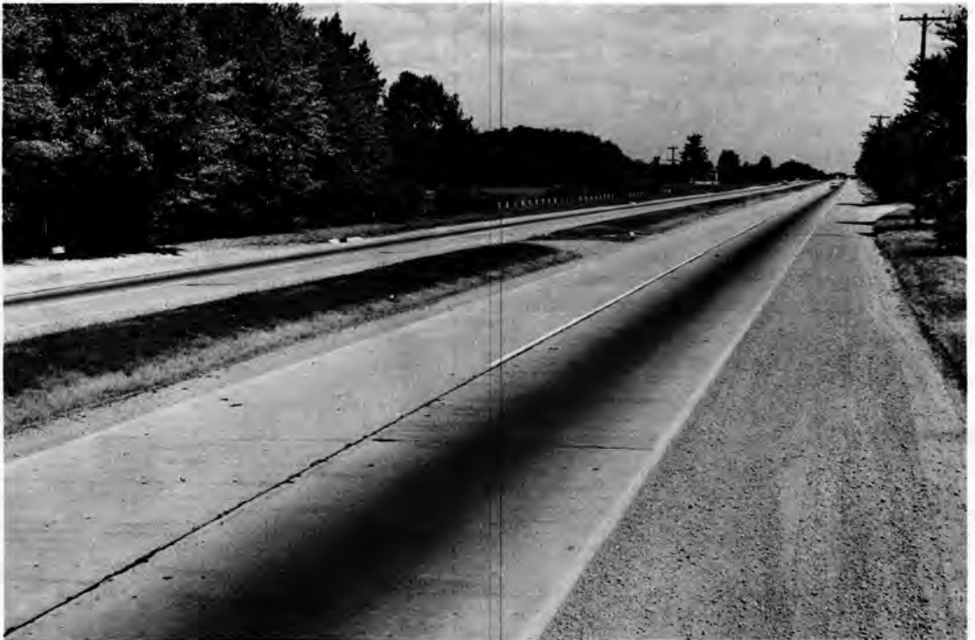
Figure 2. Eight-inch section looking north.
