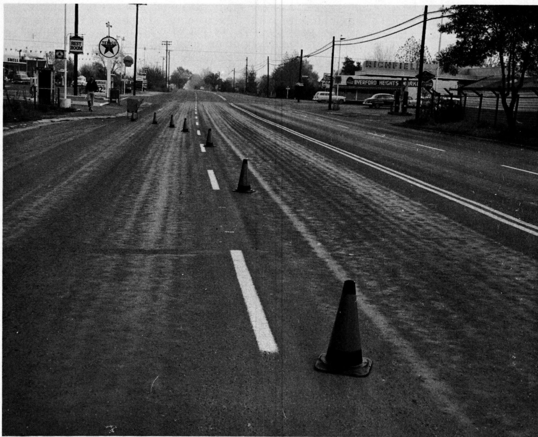
Figure 11. Appearance of seal coat three months after construction, Distributor C.
