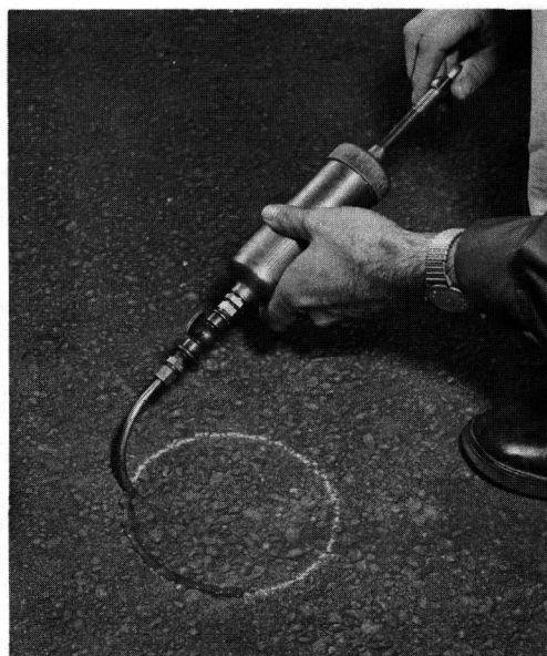
Figure 16. Forming grease ring.
