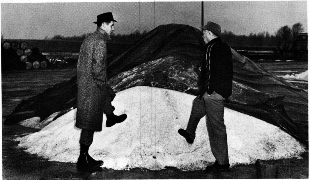
Figure 3. Maintenance personnel of the Ohio Turnpike Commission check free-flowing pile of chemical mixture after several weeks storage under tarpaulin.
