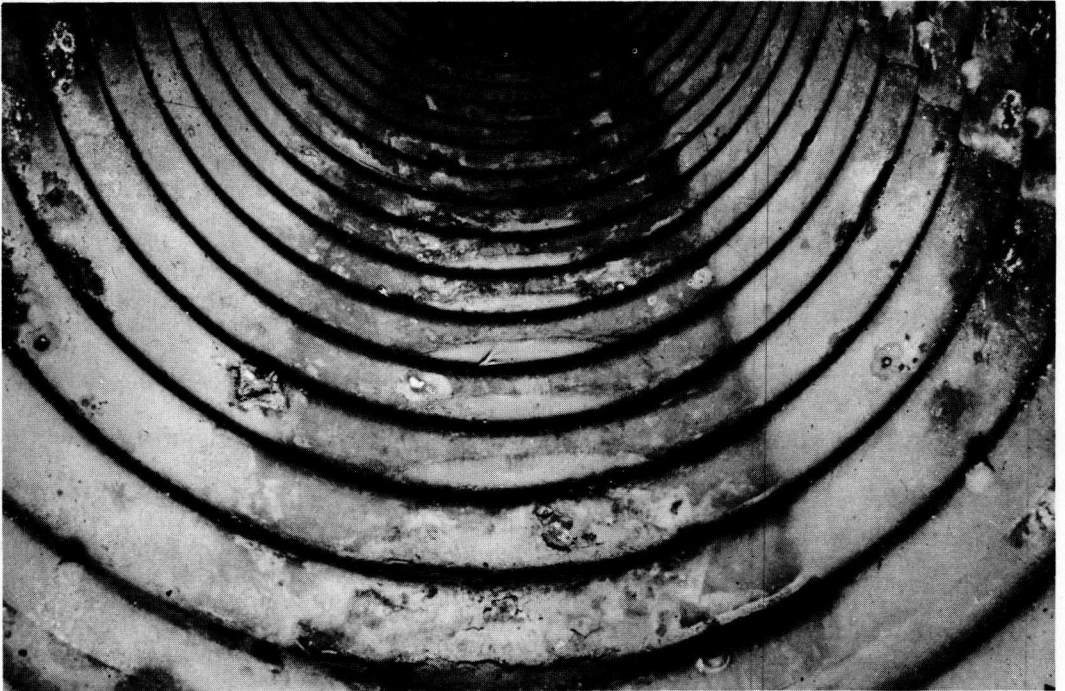
Figure 9. Depicts the appearance of the invert of a culvert located in an alkali soil area.
