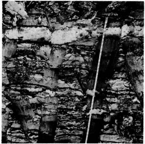
Figure 1. Small hairline ice lenses in silty soil (above). Ice lens, approximately 5 in. thick, in silty soil.
