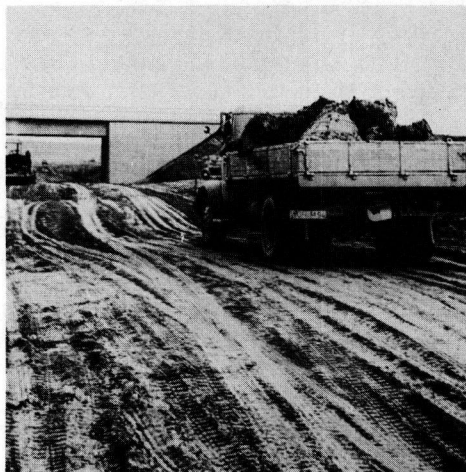
Figure 11. Lime-stabilized haul road after rainfalls.
