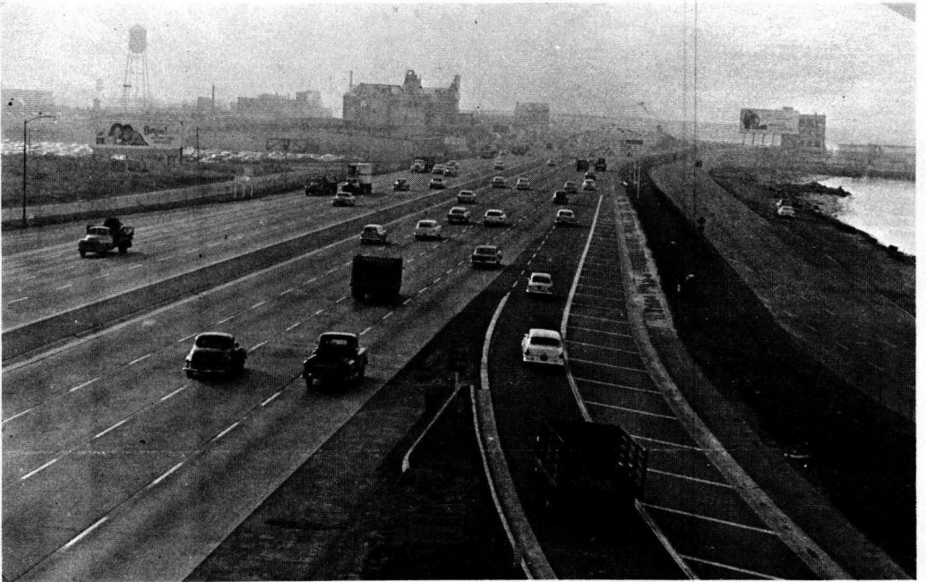
Figure 3. Test site with ramp curb offset shoulder width (in this case 8 ft from freeway pavement).
