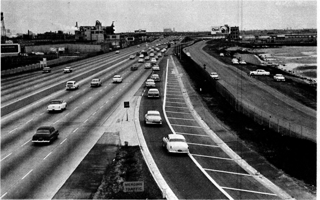
Figure 2. Test site with ramp curb encroaching on shoulder (2 ft from edge of freeway pavement).
