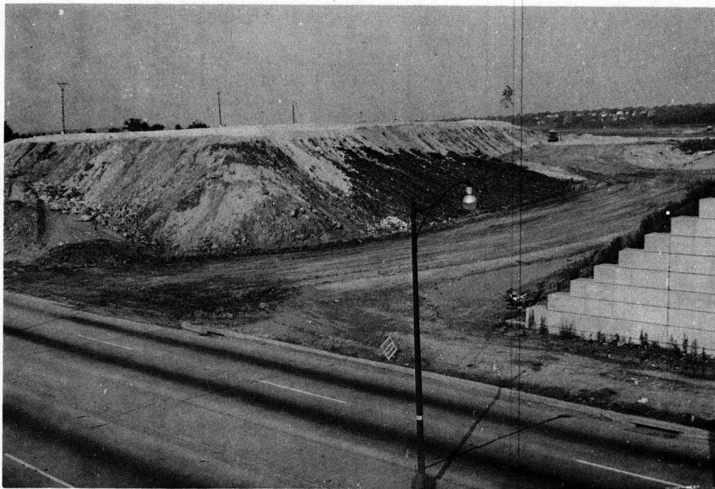
Figure 16. Station 325—embankment and surcharge.
