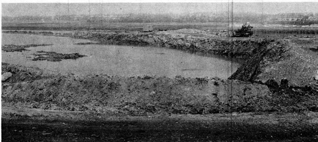
Figure 13. Station 360—area of unsuitable material.
