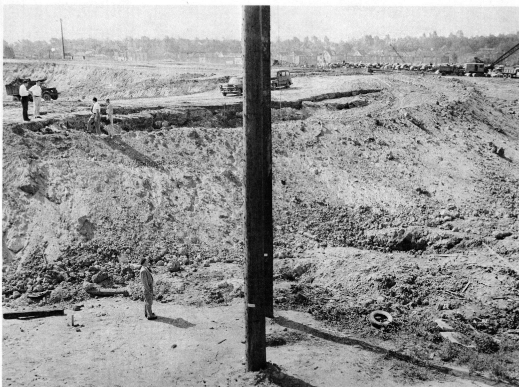
Figure 12. Off-ramp slide failure.
