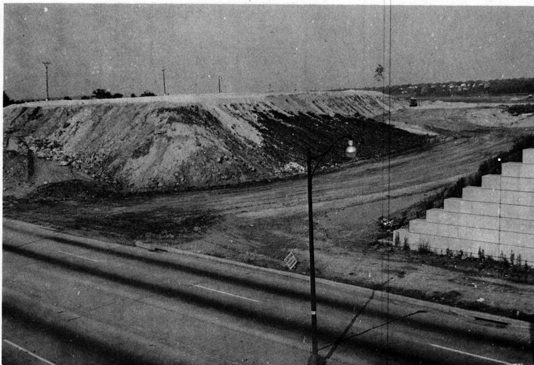
Figure 16. Station 325—embankment and surcharge.
