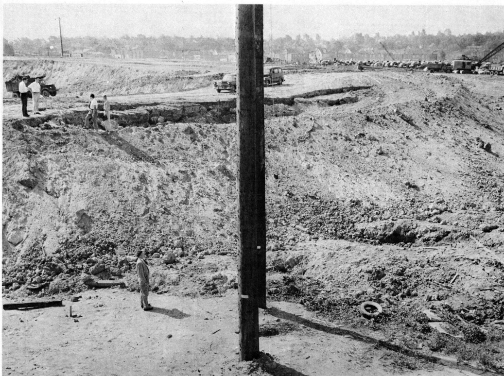
Figure 12. Off-ramp slide failure.
