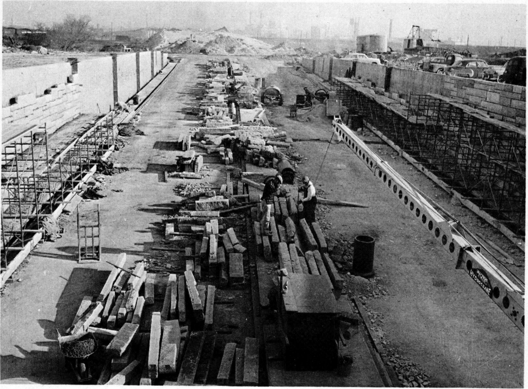
Figure 8. Open ramp near north portal of tunnel.
