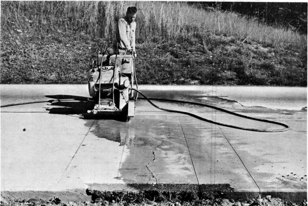
Figure 11. Sawing concrete to be removed.
