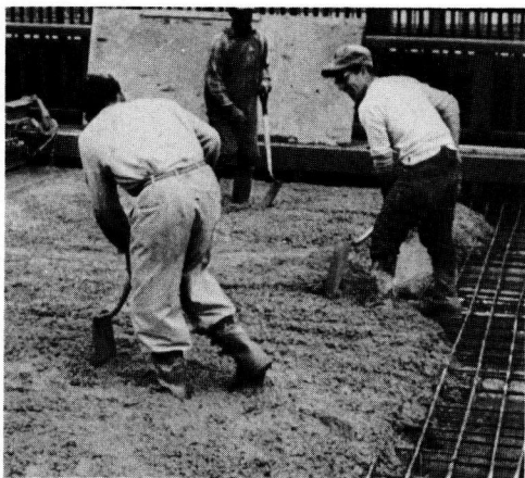
Figure 7. Spreading concrete manually.
