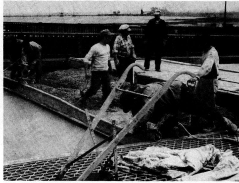
Figure 8. Vibrating screed.
