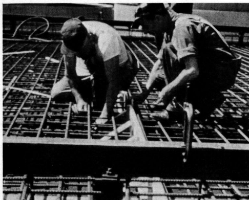
Figure 5. Placing a bulkhead.
