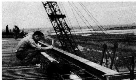
Figure 4. Checking camber.
