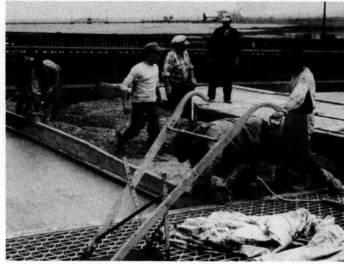
Figure 8. Vibrating screed.
