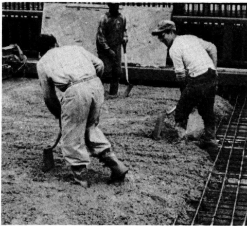
Figure 7. Spreading concrete manually.
