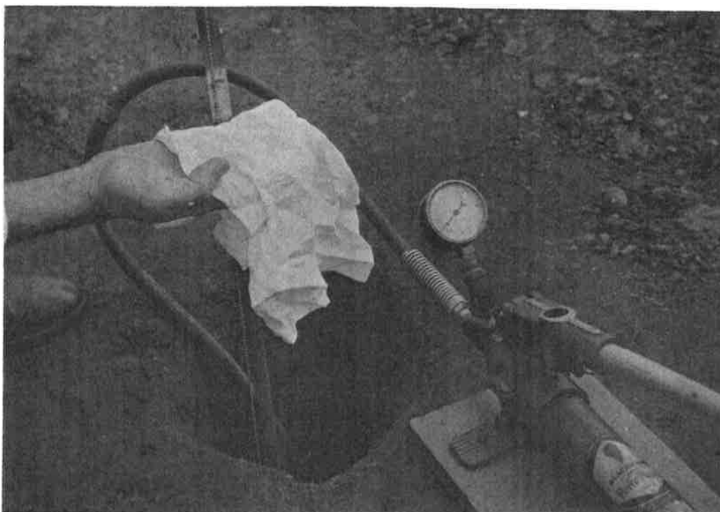
Figure 3. Device installed and under preload deflection.
