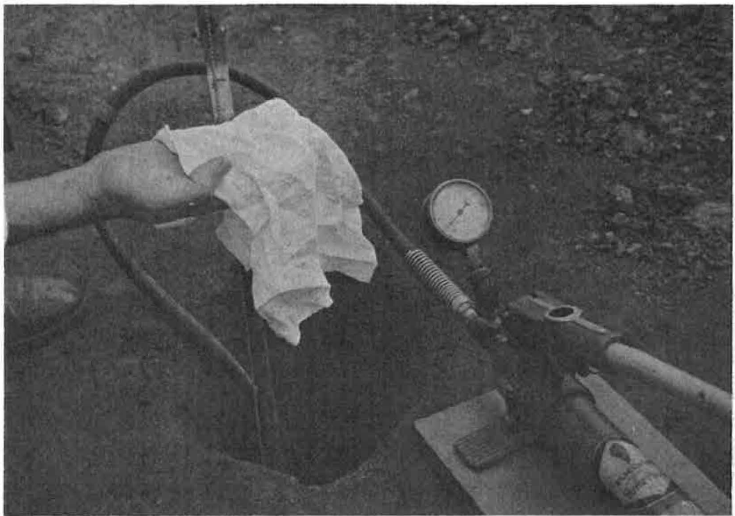
Figure 3. Device installed and under preload deflection.
