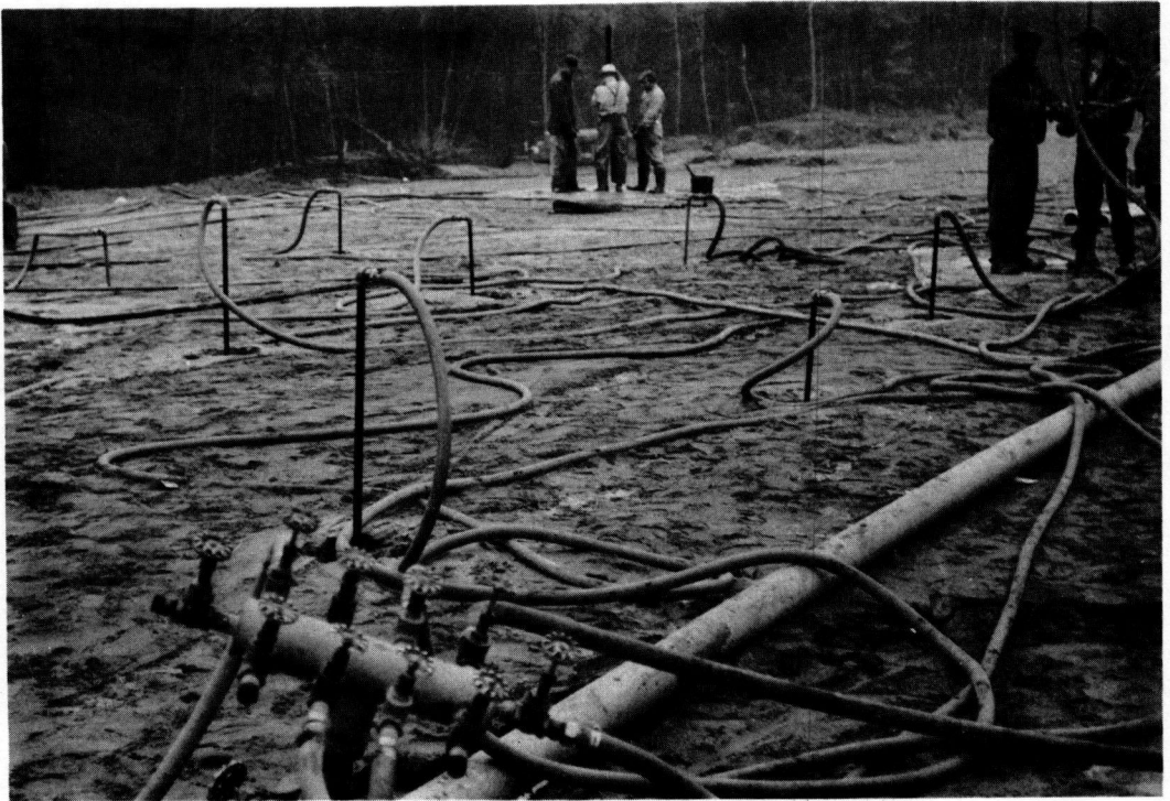
Figure 5. Jet pattern and distribution setup.
