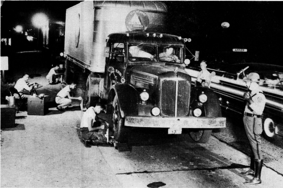
Figure 15 - Loadometer Party at Work in Pennsylvania. Simultaneous Weighing of Three Wheels. (Print furnished by Pennsylvania State Highway Department.)
