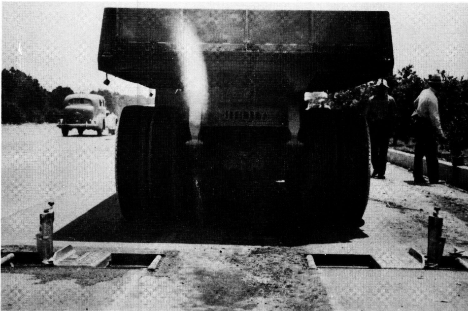
Figure 16 - New-type Loadometer Installed in Shallow Pit for Weighing Wheel Loads at Ground Level. Route U. S. 60, West Corina, California. (Print furnished by Bureau of Public Roads.)
