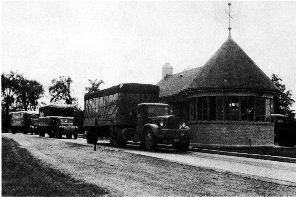
Figure 12 - Scale House in Operation on U. S. 24 near Erie, Monroe County, Michigan. (Print furnished by Michigan State Highway Department.)
