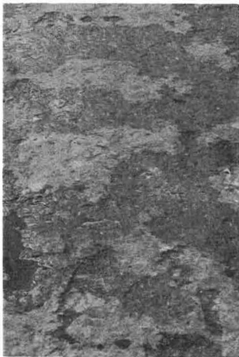
Figure 3. Typical scaled and polished concrete deck surface.
