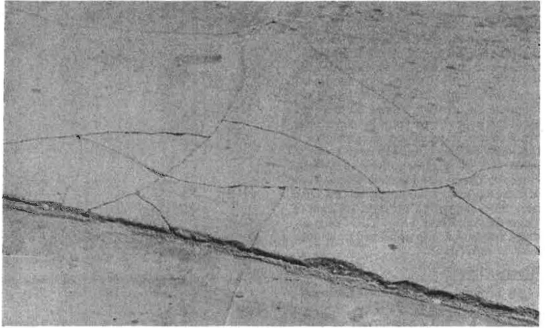
Figure 10. Extensive cracking and loose latex mortar on east end of Lane F after one winter (April 1958).
