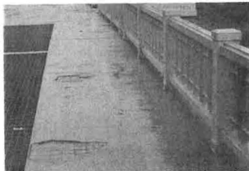
Figure 13. Newly spalled areas in north sidewalk, some adjacent to patches.
