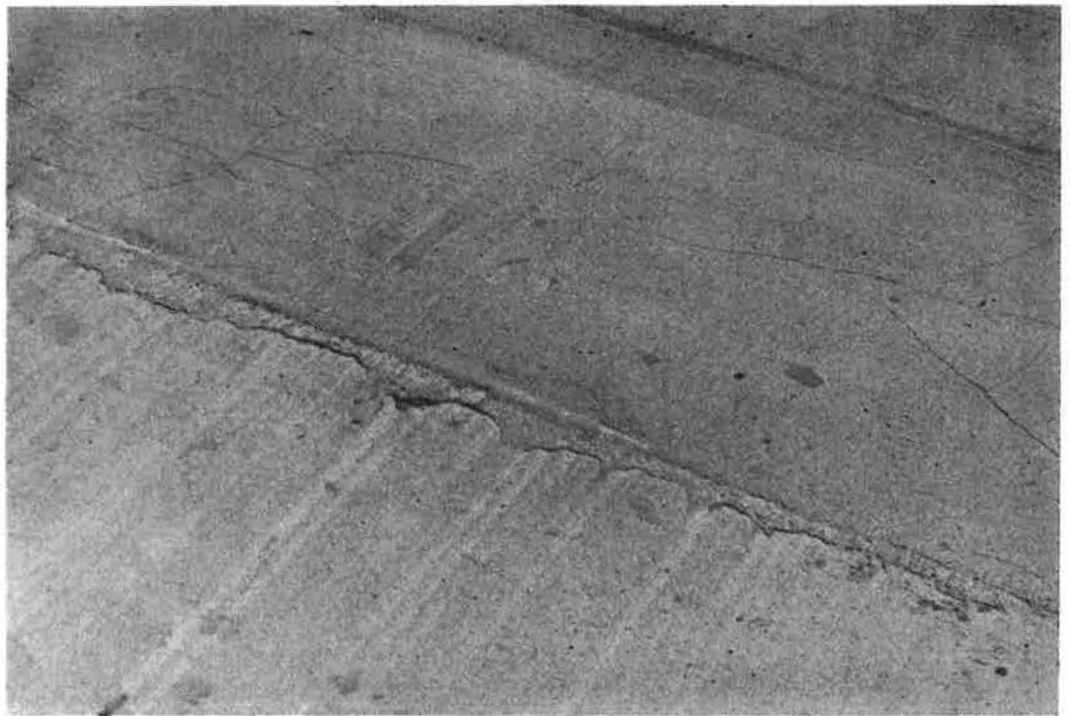
Figure 11. Cracking and loose mortar in west end of Lane D after one winter (April 1958).
