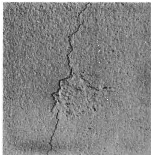
Figure 8. Shrinkage crack adjacent to sand-cement lump.
