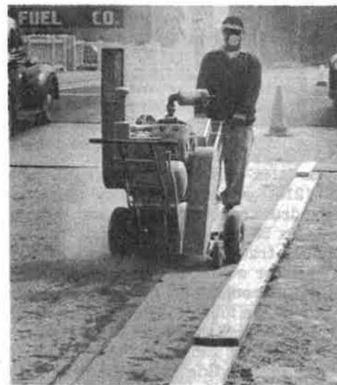
Figure 4. Cutting machine used to remove minimum of \frac{1}{2} in. of scaled concrete.
