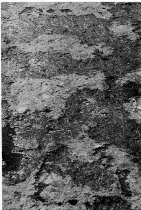
Figure 3. Typical scaled and polished concrete deck surface.
