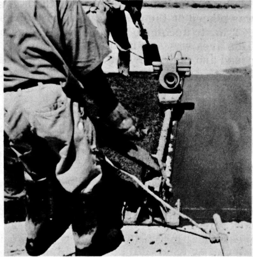
Figure 7. Hand-operated vibrating screed used at Standiford Field, Louisville,
