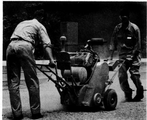
Figure 2. Tennant machine used for cleaning joints and grinding surface.
