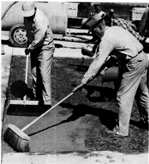
Figure 4. Spreading bonding grout.
