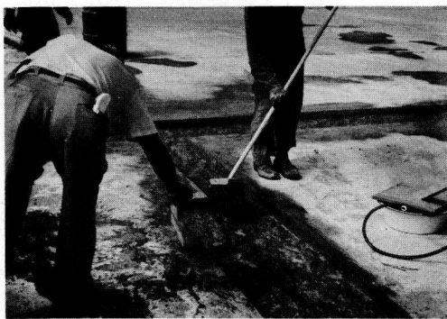
Figure 10. Prepared patch receiving acid treatment. Note improvised acid dispenser at right.
