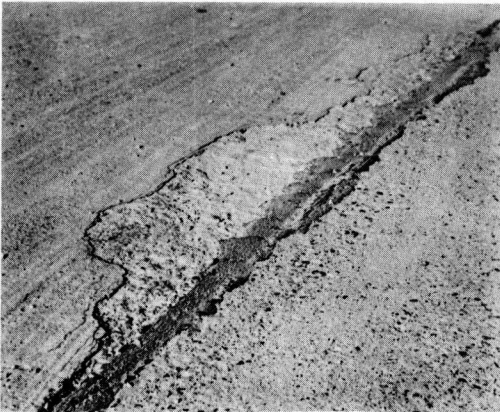
Figure 1. Scaled and raveled pavement at Selfridge Air Force Base.
