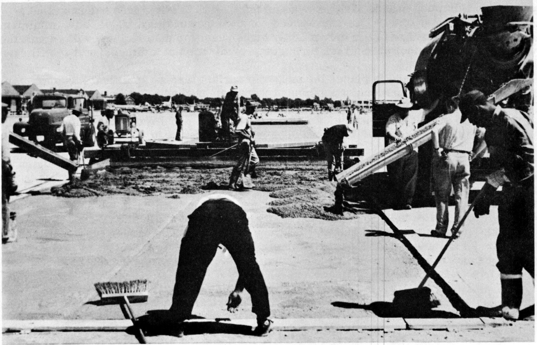
Figure 5. Concrete delivered to both sides of paving lane by transit mixers.
