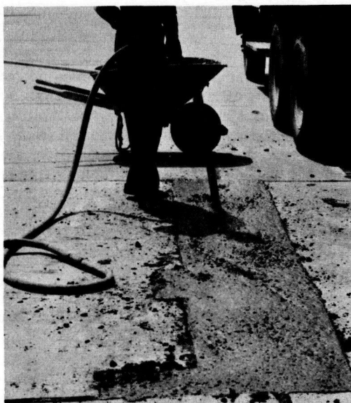
Figure 12. Hand vibrator used to consolidate concrete in patch.
