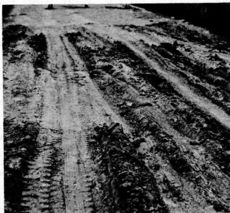
Figure 6. Condition of Highway 14 at Holmwood during the winter of 1958.
