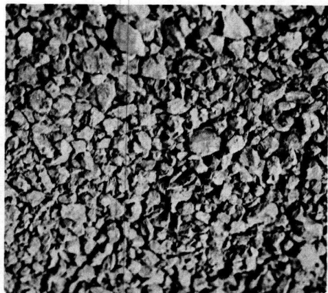
Figure 11. Mixed and pulverized soil-lime before compaction after the second application.
