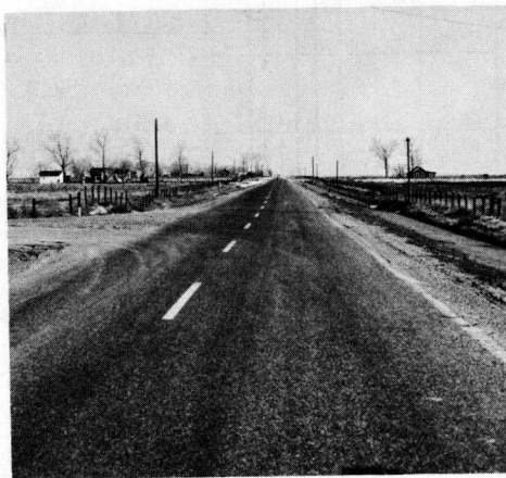
Figure 12. The finished road after it was covered with three-course bituminous treatment.
