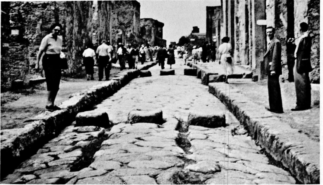
Figure 2. A street in Pompeii showing stepping stones and grooves worn by chariot wheels.
