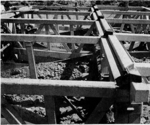
Figure 3. Windrower section of subgrader in operation.
