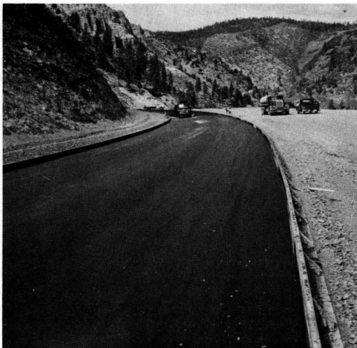
Figure 13. Subgrade in place—ready for curing seal.
