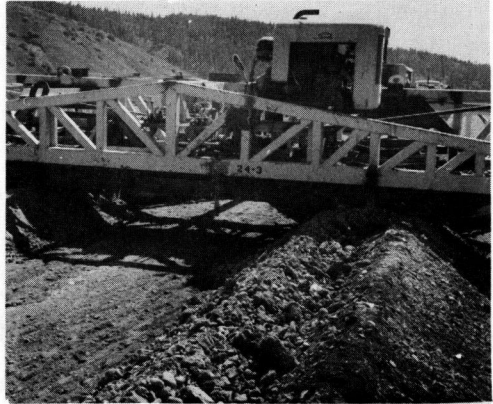
Figure 4. Dual windrows shaped by subgrader.
