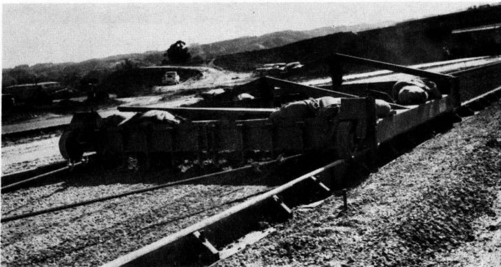
Figure 5. Cement-treated subgrade—windrow machine.
